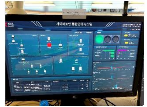
[Network monitoring system]
